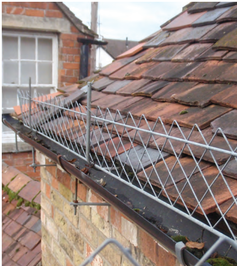
It is recommended to use at least 4 brackets per 2 metre length of snowguard
