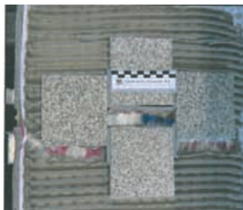
Crack widening and total rupture of decoupling
